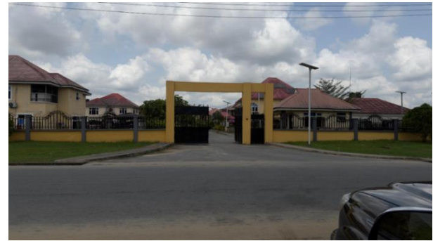
Plate 4: New Commissioners' Quarters Controlled Entrance with Defined Gate and Perimeter Fencing, Enhancing Access Control
