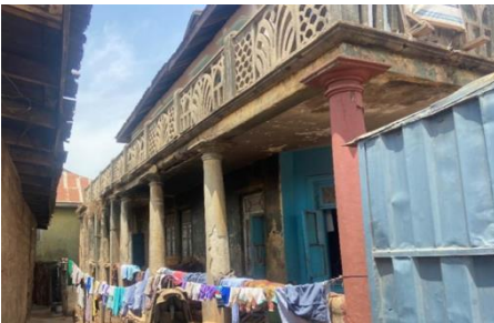
Plate 2: Right Side View of the Historic Building
