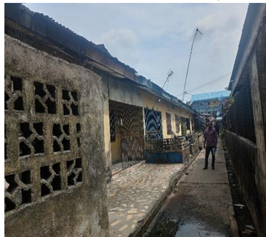
Figure 4: Building Condition in the Study
