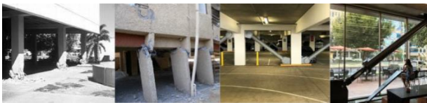
Figure 1. Collapse of structures due to the soft ground effect (left) dampers with acceptable structural and aesthetic requirements (right)
