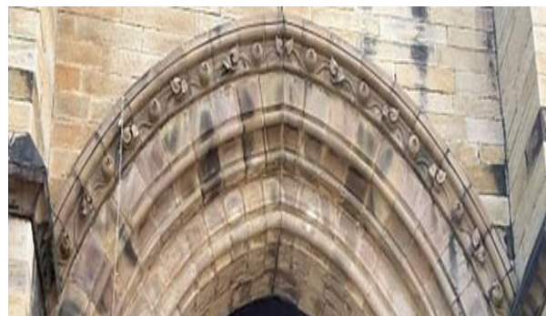
Figure 20 The entrance is marked by a deeply recessed pointed arch, composed of multiple concentric orders, particularly notable feature is the archivolt ornamentation, with a continuous floral motif carved in relief.
