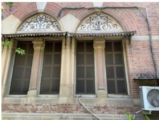
Figure 3 Segmental arches and embellished with wrought iron floral grilles, which are both decorative and functional.
