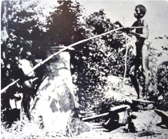
Figure 2: Local Shaft Furnace at South-Western Lake Chad. 1917. Courtesy Prof. W.J. McCaughey of Ohio State University in Sullivan, 1966
