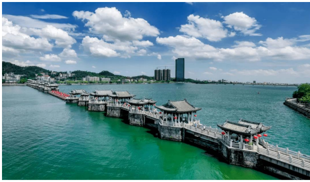
Figure 3 Landscape of Guangji Bridge
