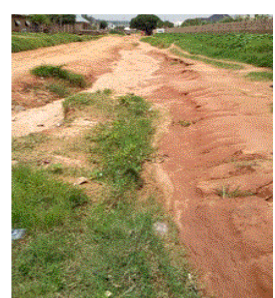
Plate 5: an eroded street at Mayo-Dassa
