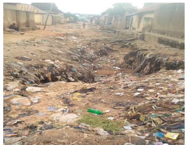
Plate 1. An affected erosion site in the Sabon-Gari. area of Jalingo
